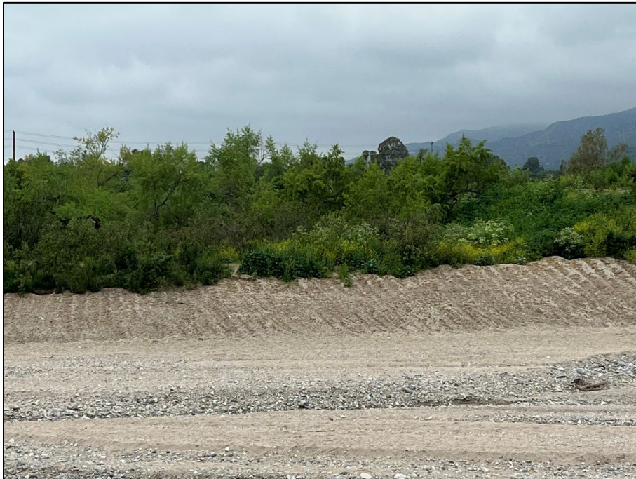
Photo 12: Overview Side Slopes
