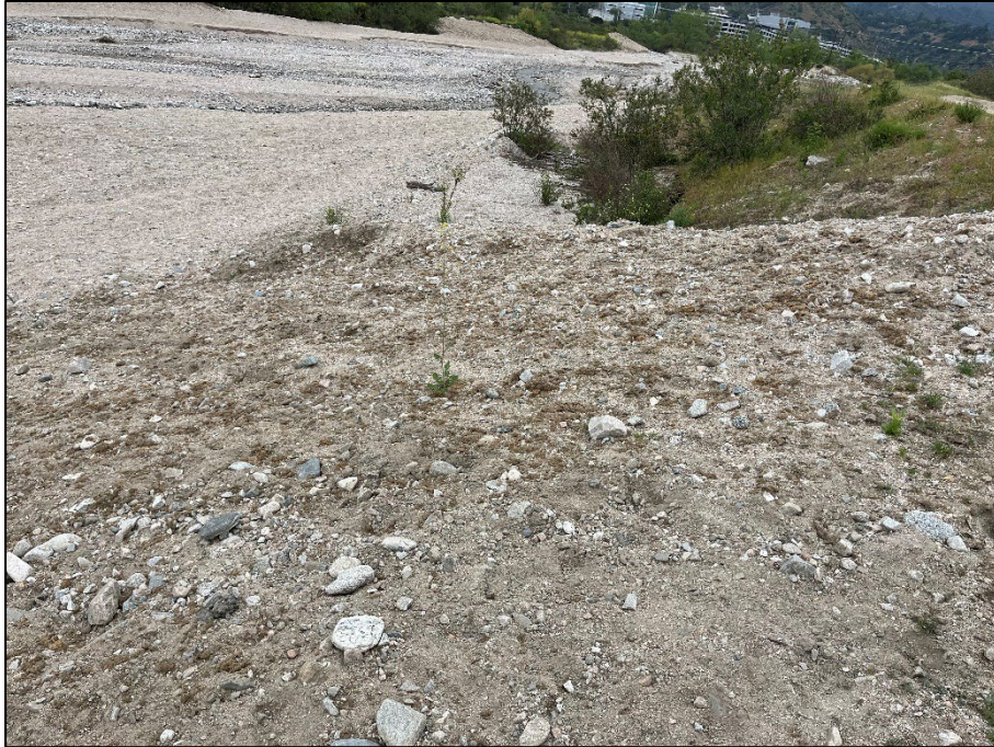
Photo 11: Overview Side Slopes
